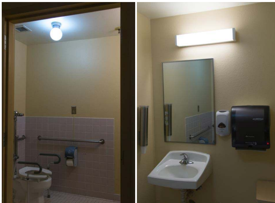
Figure 7: Incumbent bathroom lighting for both the single room and the double room. Although the physical configuration differed, the lighting for the two spaces was similar.
