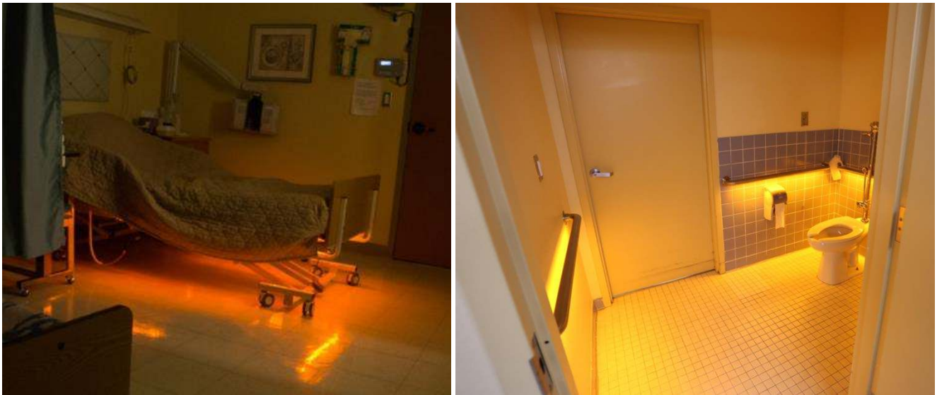
Figure 14: Nighttime lighting elements that promote good sleep hygiene. Amber rope lights were installed underneath each bed, controlled by motion sensors that would respond at night to someone getting out of bed or to a nurse entering the room (left photo). Amber LED lighting was also integrated into new handrails in the bathrooms, controlled by motion sensors to provide low-level lighting when someone entered the bathroom (right photo).
