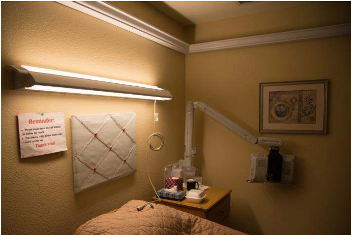
Figure 12: Wall-mounted luminaire to provide task lighting at the resident's bed. The uplight compartment is shown in its normal position, providing uplighting into the room, but it can also be tilted up to direct its light onto the bed for increased task lighting for caregivers. The downlight compartment provides task lighting for reading and is switched by the resident using the low-voltage push button switch shown at the pillow.
