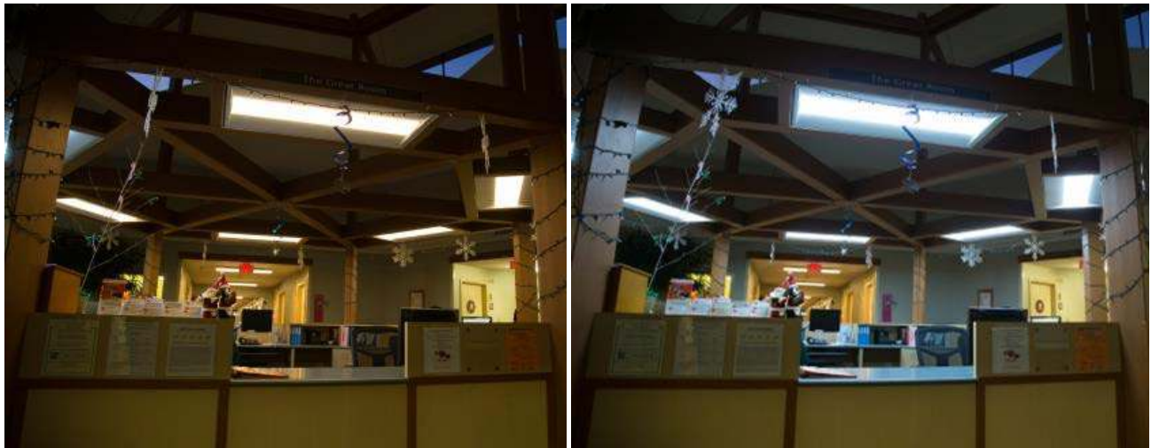
Figure 9: Tunable lighting system at the nurse station, shown at the 2700 (left) and 6500 K (right) settings. The nurses have manual control over the CCT and light output at all times for these luminaires.
