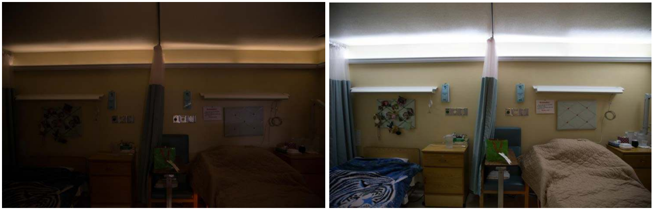
Figure 11: Ambient lighting for the resident rooms, using an LED CCT tunable cove built into a plastic wall-mounted gutter assembly. The left image illustrates the LED cove set to a dimmed level at 2400 K for nighttime use, while the right photo illustrates the system set at the morning setting of 6000 K.
