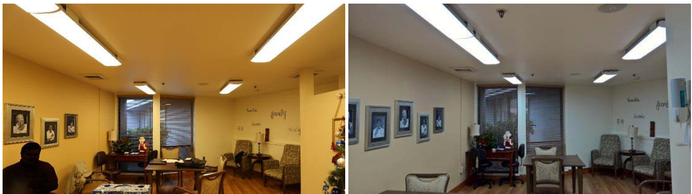
Figure 10: Tunable lighting in the family room, shown at the 2700 (left) and the 6500 K settings (right). These luminaires are manually controlled from a wall-mounted control station near the entry door from the corridor.
