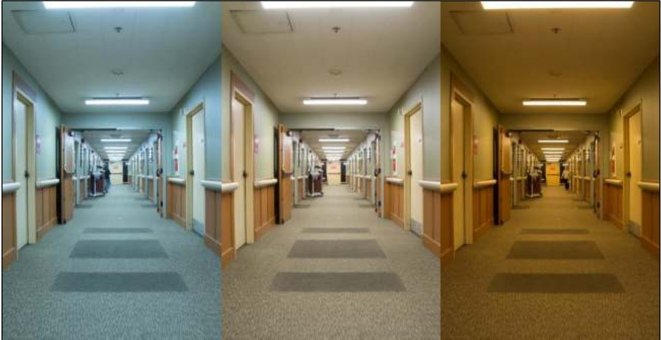
Figure 8: New tunable lighting in the corridor, illustrating the morning setting (specified as 6500 K at 66% output, left), the afternoon setting (specified as 4000 K at 66% output, center), and the nighttime setting (specified as 2700 K at 20% output, right). The corridor system operates on a programmed schedule, but the staff can override the programmed settings from a wall-mounted control station. The actual CCT at each setting is discussed in Section 4.1.
