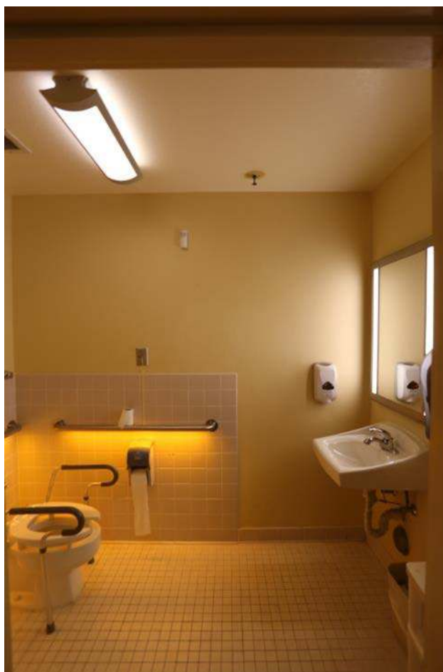
Figure 13: Bathroom lighting in the private bath for the single resident room. A mirror with integrated LED lighting was installed above the sink, and a surface-mounted LED luminaire with decorative lens was installed above the toilet area. The same luminaire types were used in the bathroom areas of the double room. The amber LED night lighting that was integrated into the railings is also shown.
